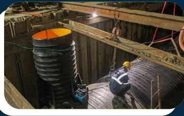
DPWH Marikina Flood Control Project Sumulong Highway
