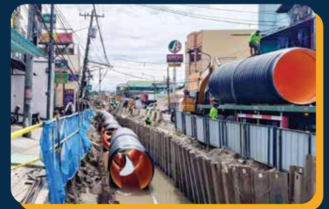
DPWH - CONSTRUCTION / REHABILITATION / UPGRADING OF DRAINAGE ROAD ALONG PANIQUI POBLACION RD PANIQUI TARLAC Pipe Installed: Covered Wall Pipes Size: ID 2,000 mm Location: Panique, Tarlac City
