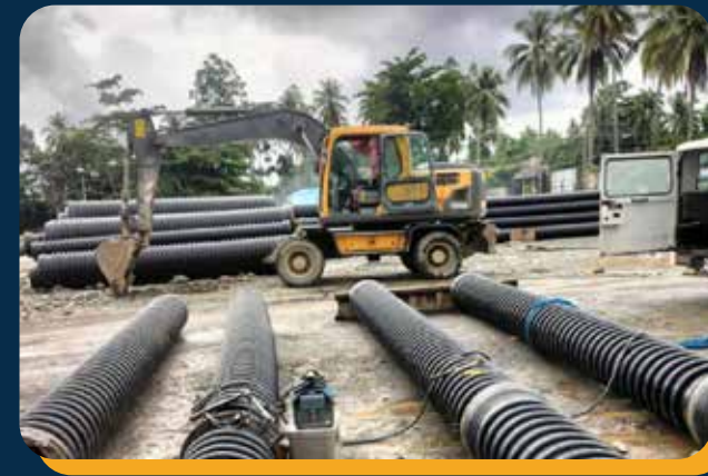
LGU - CABADBARAN PROJECT AGUSAN DEL NORTE Pipe Installed: Profiled Wall Pipe Size: ID 400, 500, 600, 800, 1,000 mm Location: Cabadbaran, Agusan del Norte
