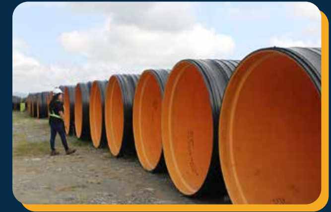
DPWH - CONSTRUCTION/ UPGRADING/REHABILITATION OF DRAINAGE ALONG NATIONAL ROADS - PRIMARY ROADS - MANUEL S. AGYAO BOULEVARD Pipe Installed: Profiled Wall Pipe Size: ID 1,800 mm Location: Tabuk City, Kalinga
