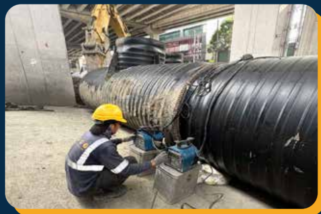
DPWH - G. ARANETA DRAINAGE SYSTEM Pipe Installed: Covered Wall Pipes Size: ID 1,500 mm Location: G. Araneta, Quezon City
