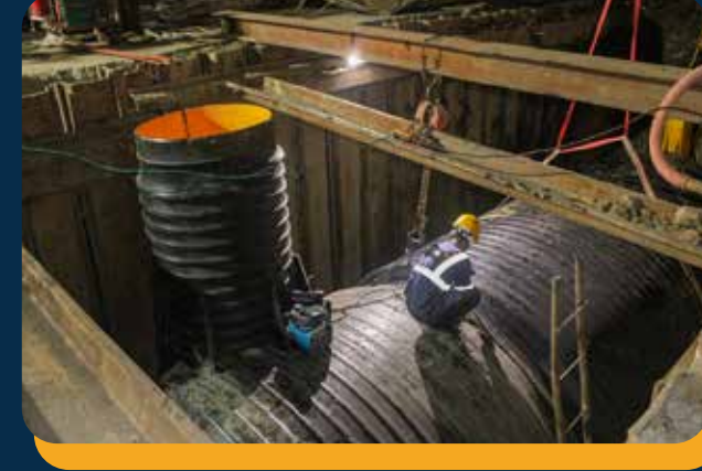
DPWH - CONSTRUCTION OF DRAINAGE SYSTEM ALONG SUMULONG HIGHWAY INCLUDING LATERALS (PHASE III) Pipe Installed: Covered Wall Pipes Pressure Rating: Gravity Size: ID 3,500 mm Location: Sumulong Highway, Marikina
