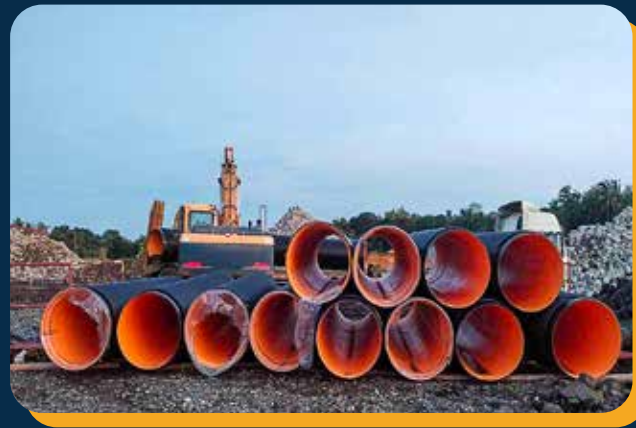
DPWH - CONSTRUCTION OF ROAD ALONG IZNART ST. AND J.M. BASA ST. WITH DRAINAGE SYSTEM Pipe Installed: Profiled Wall Pipes Size: ID 1,000 mm Location: Iloilo City
