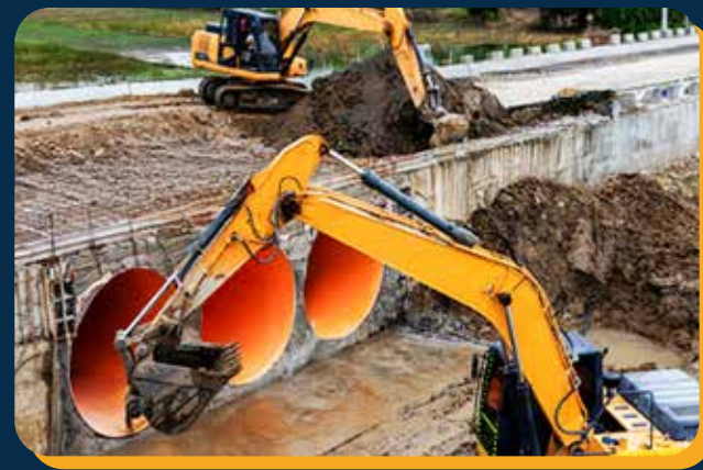
DPWH - CONSTRUCTION OF MONCADA - PANIQUI DIVERSION ROAD Pipe Installed: Profiled Wall Pipes Size: ID 3,000 mm Location: Moncada, Tarlac
