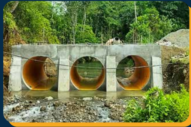
DPWH - CONSTRUCTION OF SPILLWAY IN LITTLE BAGUIO, MALAYBALAY BUKIDNON Pipe Installed: Covered Wall Pipes Size: ID 3,000 mm Location: Valencia Bukidnon
