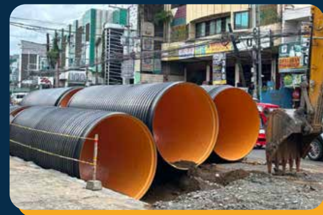
DPWH - ASSET PRESERVATION PROGRAM - CONSTRUCTION/UPGRADING/REHABILITATION OF DRAINAGE ALONG NATIONAL ROADS PRIMARY - DAANG MAHARLIKA Pipe Installed: Covered Wall Pipes Size: ID 2,000 mm Location: Maharlika Highway, Santiago City, Isabela
