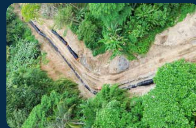
7.4 MW MALITBOG - SILO - O HYDROELECTRIC POWER PLANT Pipe Installed: Profiled Wall Pipe Ring Stiffness: SN2 Pressure Rating: 1 Bar | 2 Bar | 3 Bar Size: ID 1,500 mm Location: Malitbog, Bukidnon
