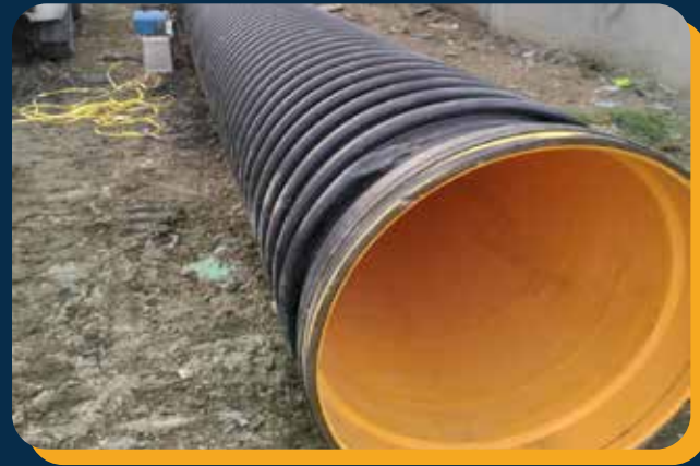
DPWH - CONSTRUCTION OF RIVERWALL ALONG TANZA DIKE, BRGY. TANZA, NAVOTAS CITY Pipe Installed: Profiled Wall Pipes Size: ID 800 mm | 96 Linear Meter Location: Tanza, Navotas City
