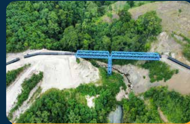
14.5MW SIGUIL HYDROELECTRIC POWER PLANT Pipe Installed: Solid & Structured Wall Pipe Ring Stiffness: SN2 Pressure Rating: Atmospheric Size: ID 2,000 mm | Length: 18 KM Location: Maasim, Siguil, General Santos, Mindanao
