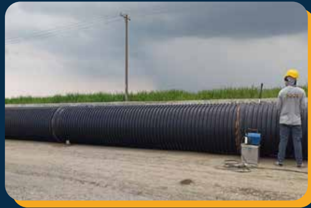
DPWH - NEW CLARK CITY ACCESS ROAD DRAINAGE PROJECT Pipe Installed: Profiled Wall Pipes Size: ID 1,000 mm Location: San Jose, Tarlac
