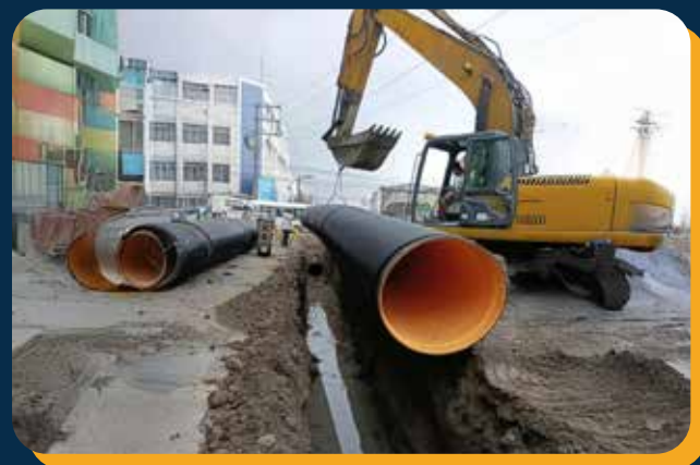
DPWH - BACOLOD CITY DRAINAGE PROJECT Pipe Installed: Profiled Wall Pipe Size: ID 1,000 mm & 1,200 mm Location: Aganan, Oton, Iloilo City
