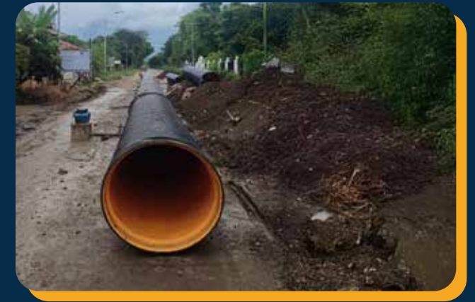
DPWH - NARRA PALAWAN DRAINAGE PROJECT Pipe Installed: Profiled Wall Pipes Size: ID 800 mm Length: 120 Linear Meter Location: Narra Palawan
