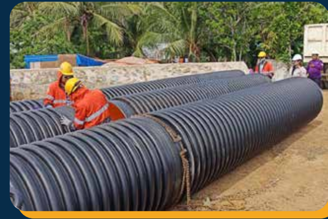
DPWH - CONSTRUCTION / MAINTENANCE OF FLOOD MITIGATION STRUCTURES AND DRAINAGE SYSTEMS Pipe Installed: Profiled Wall Pipes Size: ID 1,000 mm Location: Balud, Masbate
