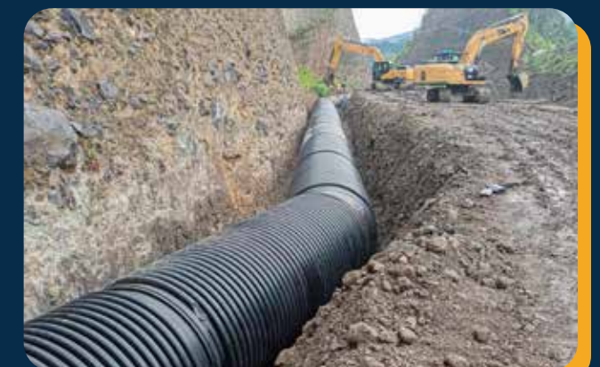
12 MW MANGIMA HYDROELECTRIC POWER PLANT Pipe Installed: Covered Wall Pipe Ring Stiffness: SN4 Pressure Rating: 2 Bar | 3 Bar | 4 Bar Size: ID 2,000 mm | Length: 6 KM Location: Mangima, Bukidnon
