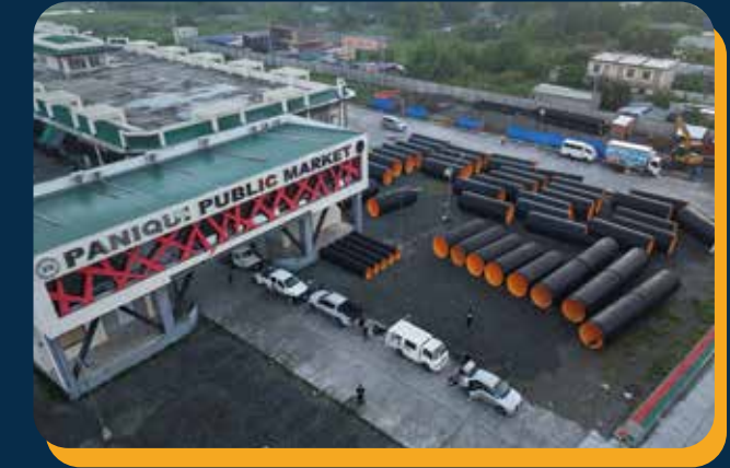
DPWH - PANIQUI DRAINAGE PHASE 2 Pipe Installed: Covered Wall Pipes Size: ID 1,000 mm & 2,000 mm Location: Paniqui, Tarlac
