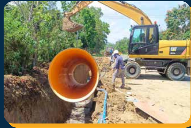
DPWH - CONSTRUCTION/UPGRADING/ REHABILITATION OF DRAINAGE ALONG BUTUAN-CDO NATIONAL ROAD - CARAGA REGION PROJECT Pipe Installed: Covered Wall Pipes Size: ID 1,000 mm & 2,000 mm Location: Butuan City, Agusan del Norte
