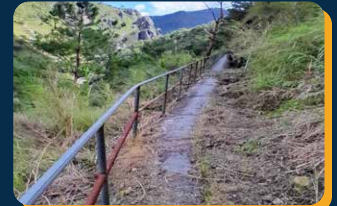
LOWER LABAY HYDROELECTRIC POWER PLANT Pipe Installed: Solid Wall Pipe Pressure Rating: 2.1 Bar Size: ID 1,400 mm Location: Bakun, Benguet
